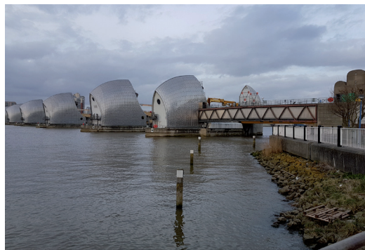
Fig 5.6a Thames Barrier, sluice in River Thames, England
