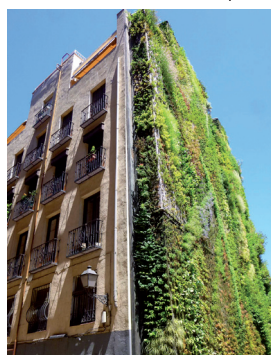
Fig 5.4 Building with vertical greening viii
