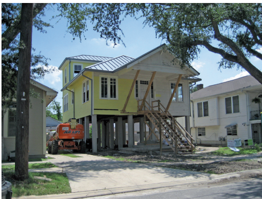
Fig 5.7 Flood resilient house
